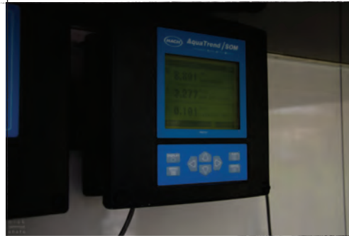
Onboard turbidity readers indicate when the water filtration process meets safe drinking water standards.
